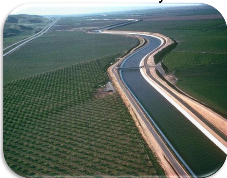
State Water Project
