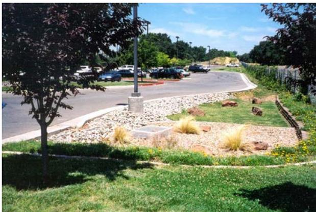
**Sand filters connected to impervious surfaces**
