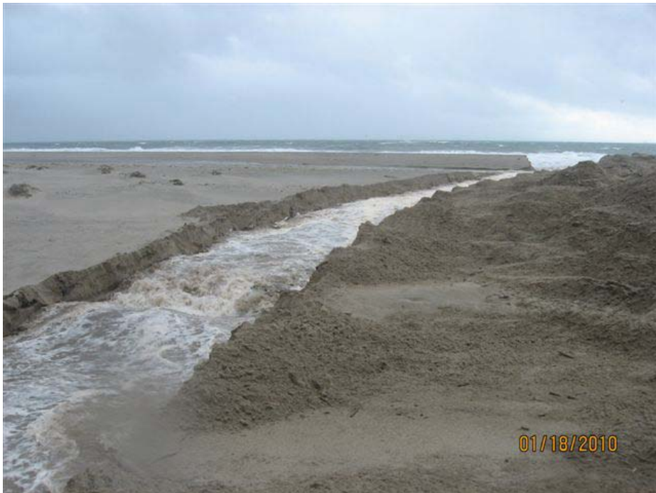
Photo 10: View south along the excavated breach channel toward its junction with the ocean.
