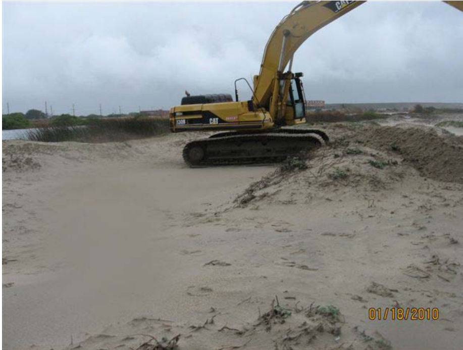
Photo 7: View southeast toward the excavator as it approached the lagoon.
