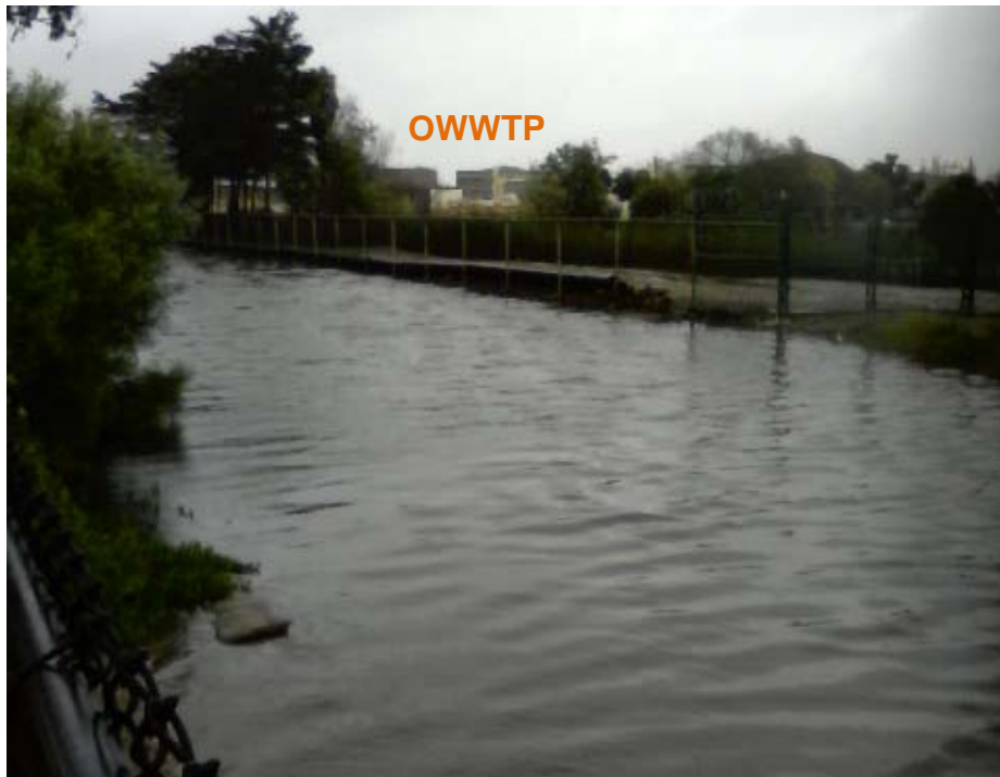
Photo 4: View northeast toward JSD, which was close to overtopping its banks and contributing additional floodwaters to the OWWTP, already flooded by OID.
