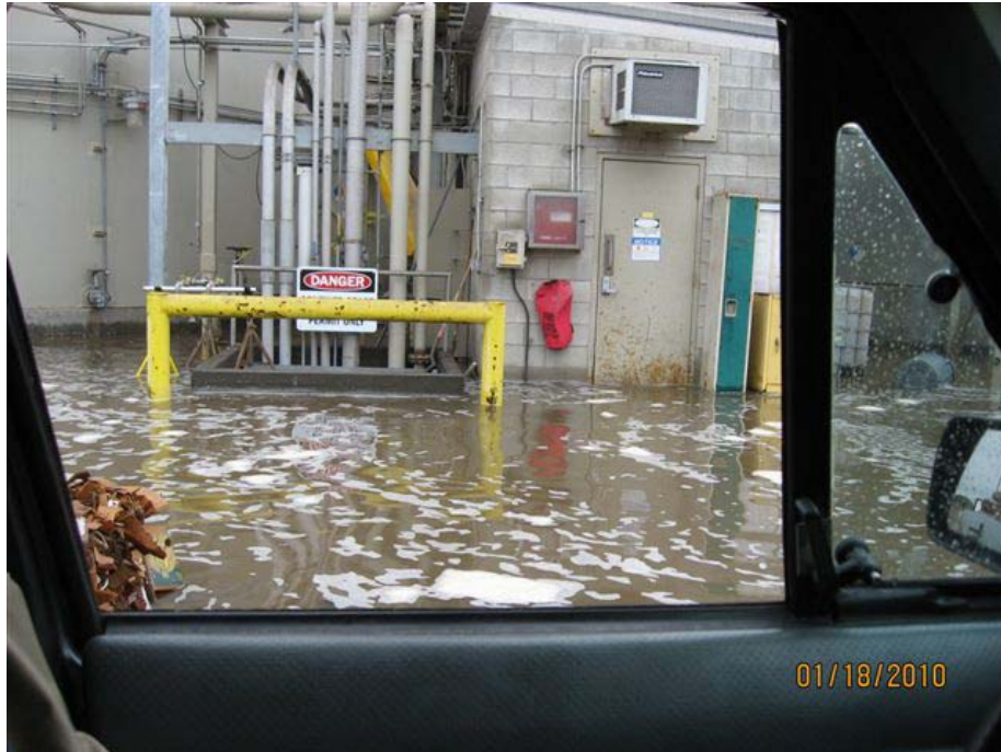
Photo 1: Flooding at the IPP threatened its electrical systems and employees attempting to protect the facility.
