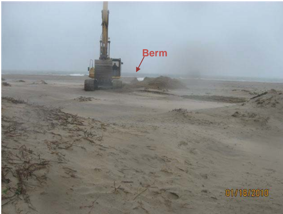
Photo 6: Excavation of the emergency breach channel, view southwest toward the Pacific Ocean. Work began at the ocean shoreline and progressed toward the lagoon shoreline.
