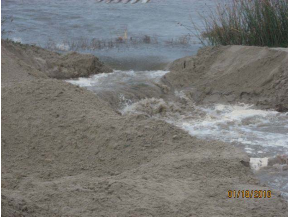
Photo 9: View northeast toward the junction of the excavated breach channel and the lagoon. This surface water release alleviated flooding at the IPP, OWWTP, Surfside III community, and streets within the City of Oxnard.
