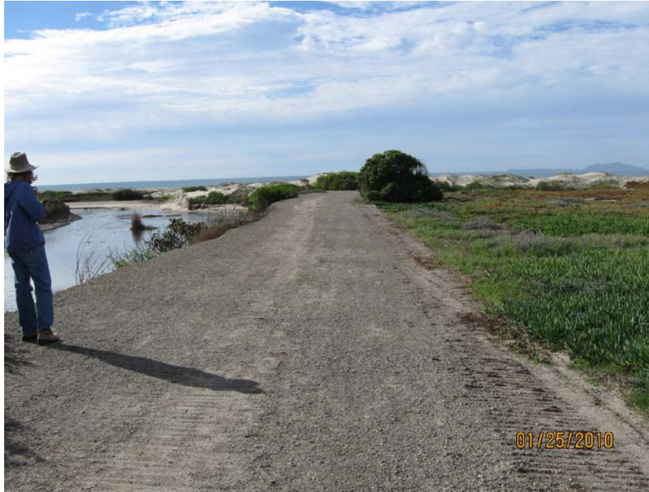
Photo 13: View southwest along the portion of the excavator access route on existing dirt road adjacent to the JSD. This and all subsequent photos were taken one week after the emergency breach action.
