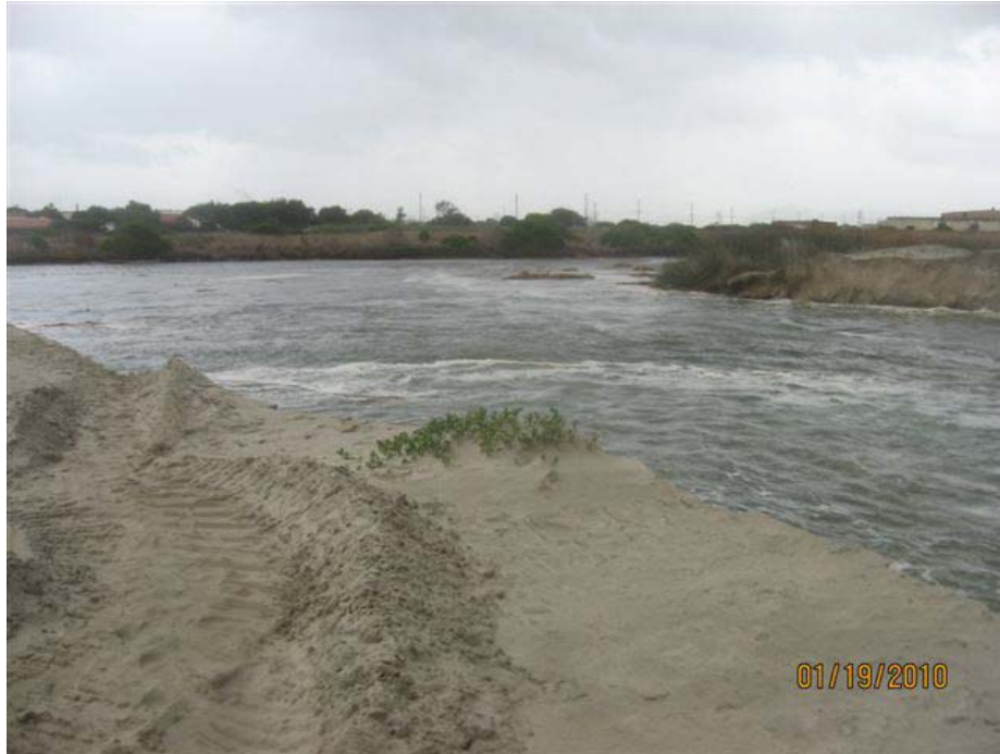
Photo 11: This photo was taken the day after the emergency action and shows that flow exiting the lagoon had considerably widened the excavated breach channel. View northeast toward the lagoon.
