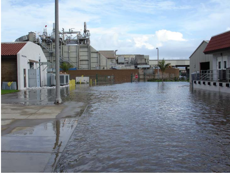
Photo 3: View east toward Perkins Road and the IPP. The structure on the left whose entrance is protected by sandbags is the Main Electrical Building for OWWTP. Inundation of equipment in this building would have caused release of untreated sewage to residential, commercial, lagoon, beach, and ocean areas.
