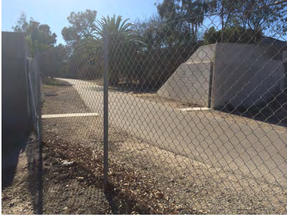
Figure 1. VR-1 Levee opening in the northern levee extension at Ventura River Bike Trail (stop-logs are used during the rainy season to close the gap) – looking south
