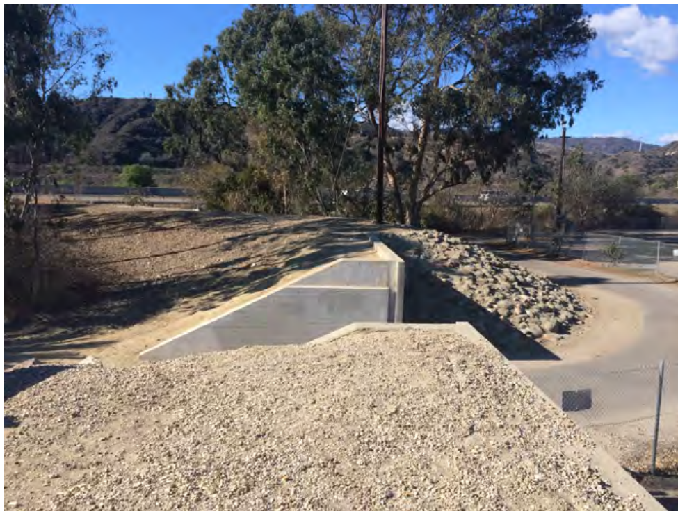
Figure 2. VR-1 Levee opening in the northern levee extension at Ventura River Bike Trail – looking west from the top of the levee
