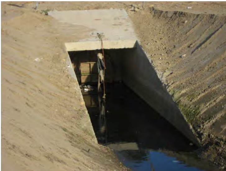
Ventura River Levee, From Ocean to Canada de San Joaquin. (Photo No. M2) - Damaged concrete on 72" RCP headwall (riverward side)
