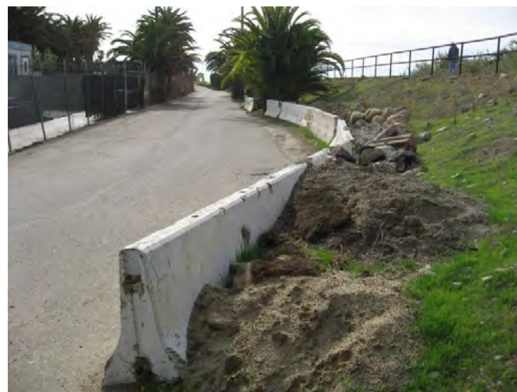
Ventura River Levee, From Ocean to Canada de San Joaquin. (Photo No. M23) – K-rails and debris along levee toe, looking d/s (landward side)
