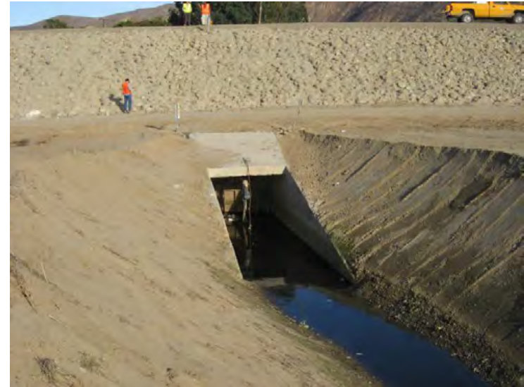
Ventura River Levee, From Ocean to Canada de San Joaquin. (Photo No. P11) - 72" RCP with flap Gate, Ramona Drain (riverward side)
