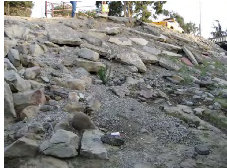
Ventura River Levee, From Ocean to Canada de San Joaquin. (Photo No. M27) – Dumped debris over levee embankment (riverward side)
