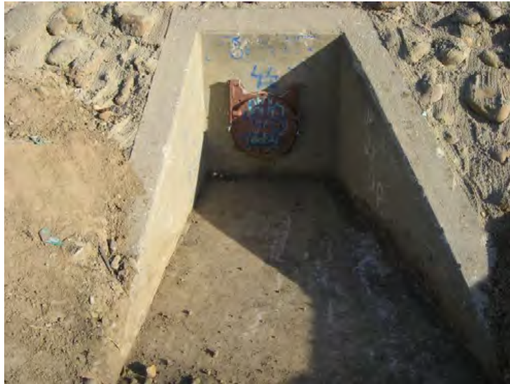
Ventura River Levee, From Ocean to Canada de San Joaquin. (Photo No. P9) - 24" CMP with flap gate, FWY #3 Drain (riverward side)
