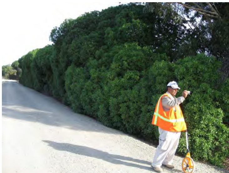
Ventura River Levee, From Ocean to Canada de San Joaquin. (Photo No. M14) - Vegetation within 15' of levee toe, looking d/s (landward side)
