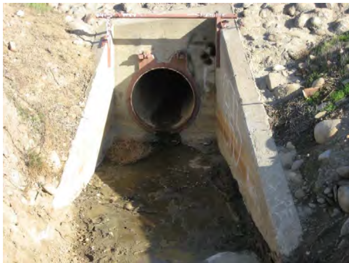
Ventura River Levee, From Ocean to Canada de San Joaquin. (Photo No. P6) - 48" RCP with missing flap gate being repaired on 12/10/08, Stanley Drain (riverward side)
