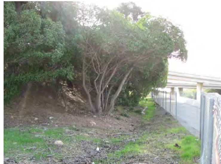
Ventura River Levee, From Ocean to Canada de San Joaquin. (Photo No. M20) - Vegetation within 15' of levee toe, looking u/s (landward side)
