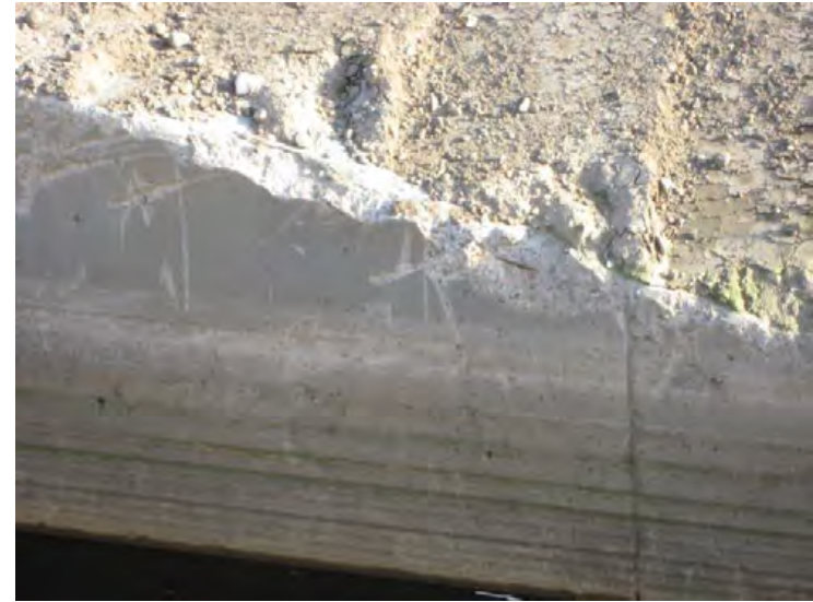
Ventura River Levee, From Ocean to Canada de San Joaquin. (Photo No. M3) - Damaged concrete on headwall with rebar exposed (riverward side)
