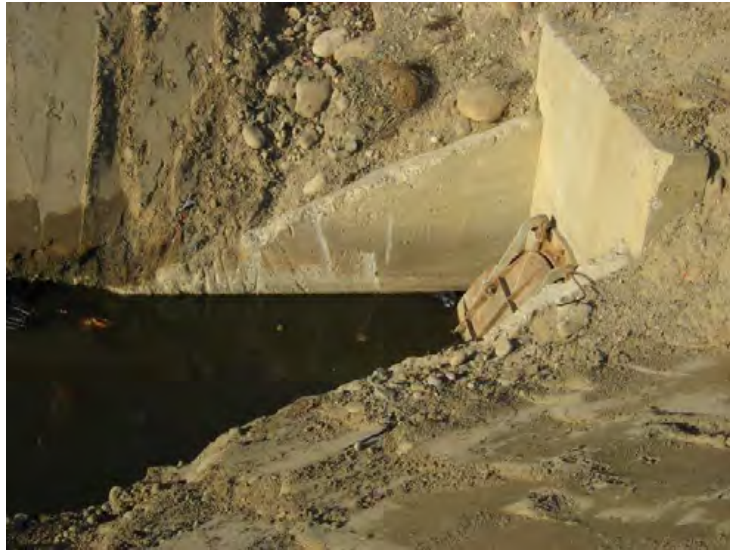
Ventura River Levee, From Ocean to Canada de San Joaquin. (Photo No. M5) - Damaged concrete on headwall with rebar exposed (riverward side)
