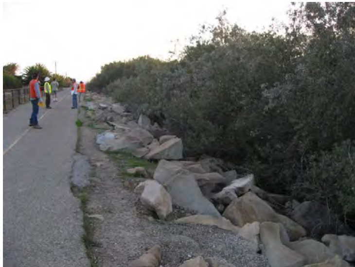
Ventura River Levee, From Ocean to Canada de San Joaquin. (Photo No. M6) - Vegetation within 15' of levee toe, looking d/s (riverward side)
