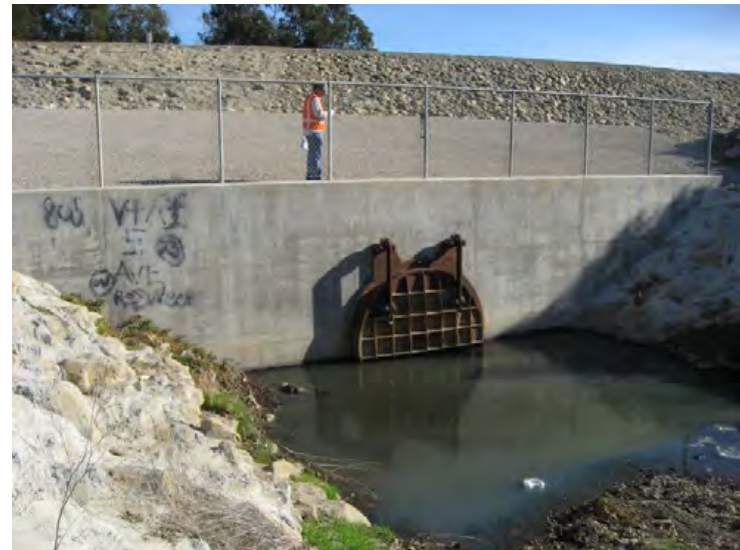
Ventura River Levee, From Ocean to Canada de San Joaquin. (Photo No. P4) - 90" RCP with flap gate, New Dent Drain (riverward side)
