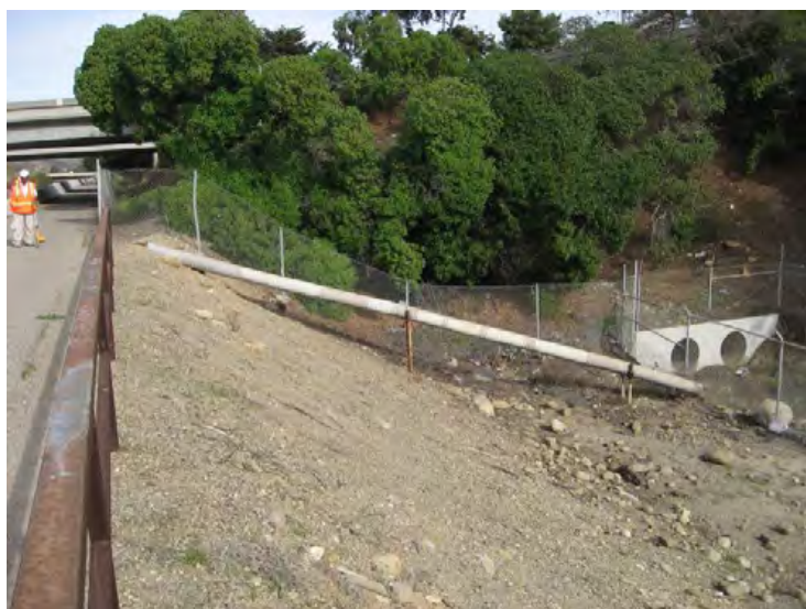
Ventura River Levee, From Ocean to Canada de San Joaquin. (Photo No. M21) – Vegetation within 15' of levee toe, looking u/s (landward side)
