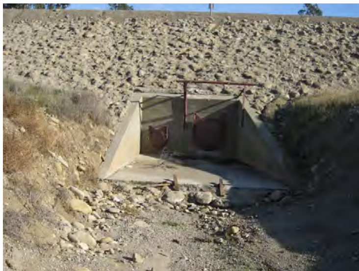
Ventura River Levee, From Ocean to Canada de San Joaquin. (Photo No. P5) - 24" & 42" CMP with flap gates, Old Dent Drain (riverward side)
