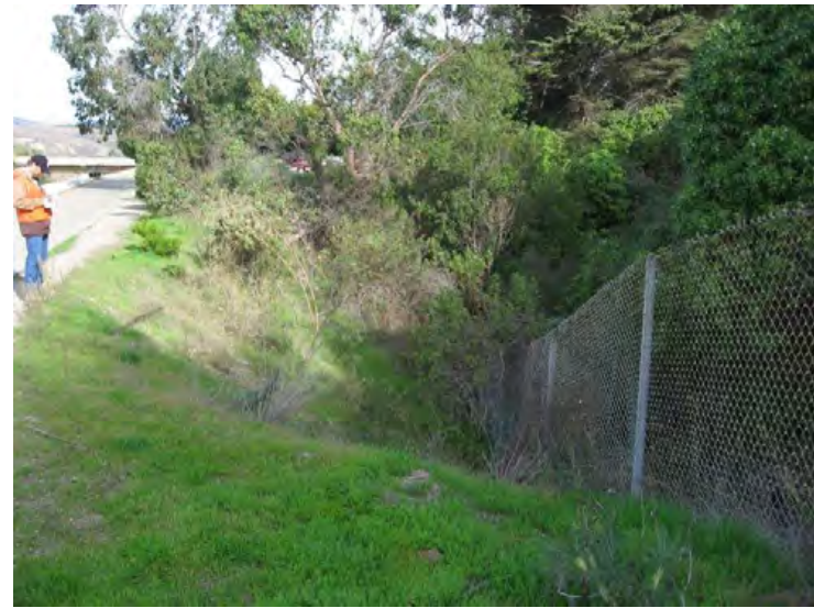
Ventura River Levee, From Ocean to Canada de San Joaquin. (Photo No. M19) - Vegetation within 15' of levee toe (landward side)
