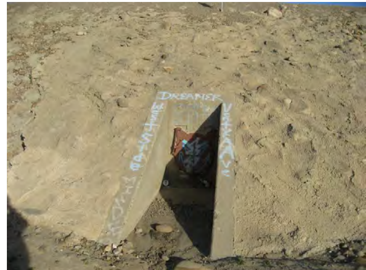
Ventura River Levee, From Ocean to Canada de San Joaquin. (Photo No. P12) - 24" RCP with flap gate, FWY #1 Drain (riverward side)
