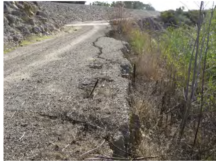
Ventura River Levee, From Ocean to Canada de San Joaquin. (Photo No. F3) – Looking d/s at low flow erosion (riverward side)
