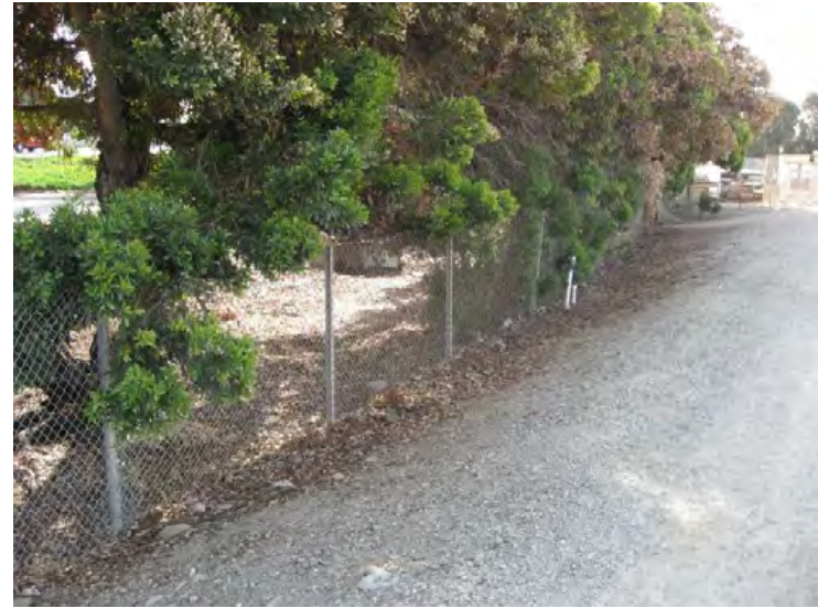
Ventura River Levee, From Ocean to Canada de San Joaquin. (Photo No. M11) - Vegetation within 15' of levee toe, looking d/s (landward side)
