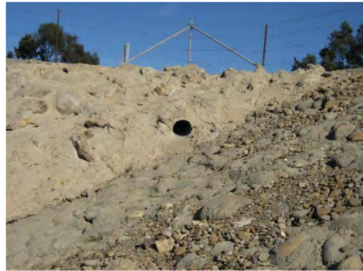
Ventura River Levee, From Ocean to Canada de San Joaquin. (Photo No. P3) - 12" CMP, drains turn out area adjacent to Hwy 33 (riverward side)
