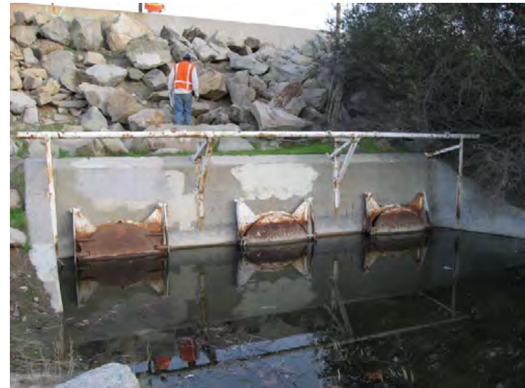
Ventura River Levee, From Ocean to Canada de San Joaquin. (Photo No. P16) - 3-48" CMP with flap gates (riverward side)
