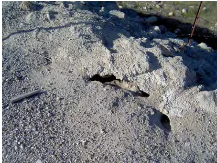
Ventura River Levee, From Ocean to Canada de San Joaquin. (Photo No. M30) – Sink holes on top of levee embankment (riverward side)
