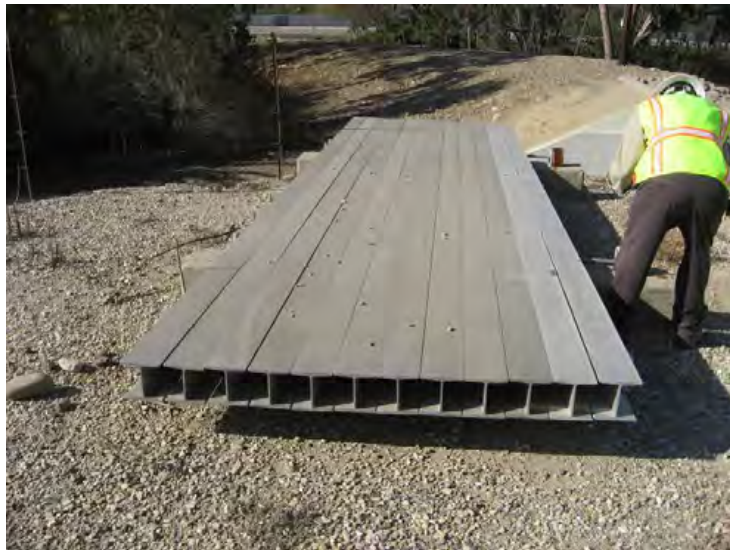
Ventura River Levee, From Ocean to Canada de San Joaquin. (Photo No. P2) - 12 beams for stop log system located on top of levee
