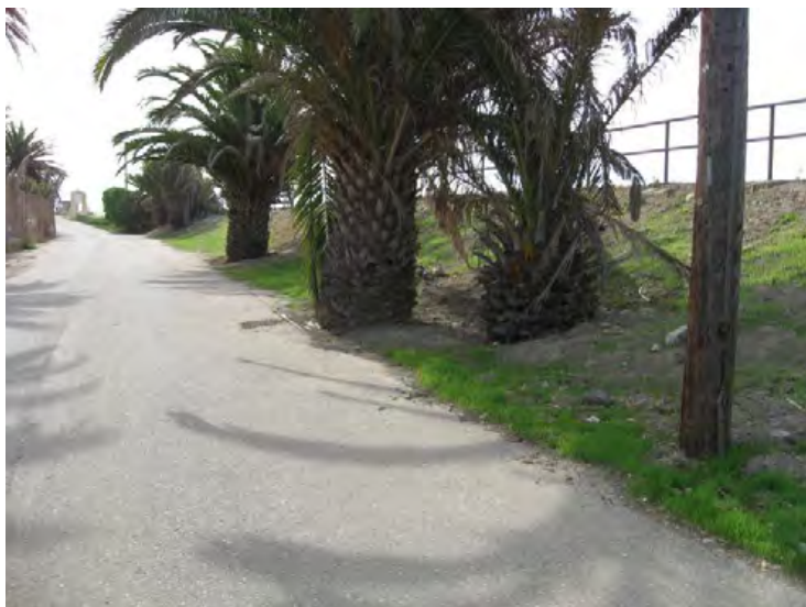
Ventura River Levee, From Ocean to Canada de San Joaquin. (Photo No. M22) - Vegetation within 15' of levee toe, looking d/s (landward side)
