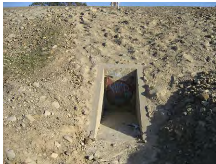
Ventura River Levee, From Ocean to Canada de San Joaquin. (Photo No. P8) - 36" Flap Gate, Vince Drain (riverward side)
