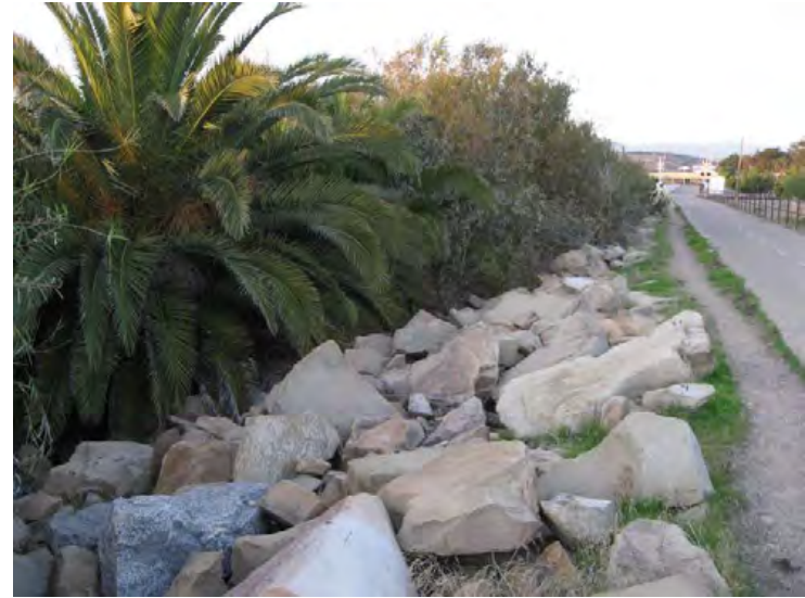
Ventura River Levee, From Ocean to Canada de San Joaquin. (Photo No. M7) - Vegetation within 15' of levee toe, looking u/s (riverward side)
