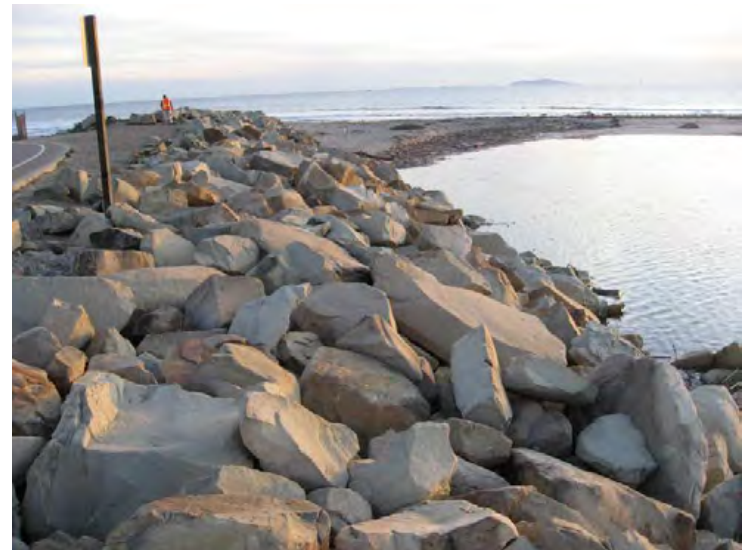
Ventura River Levee, From Ocean to Canada de San Joaquin. (Photo No. F4) – Looking d/s at ungrouted levee bank protection (riverward side)
