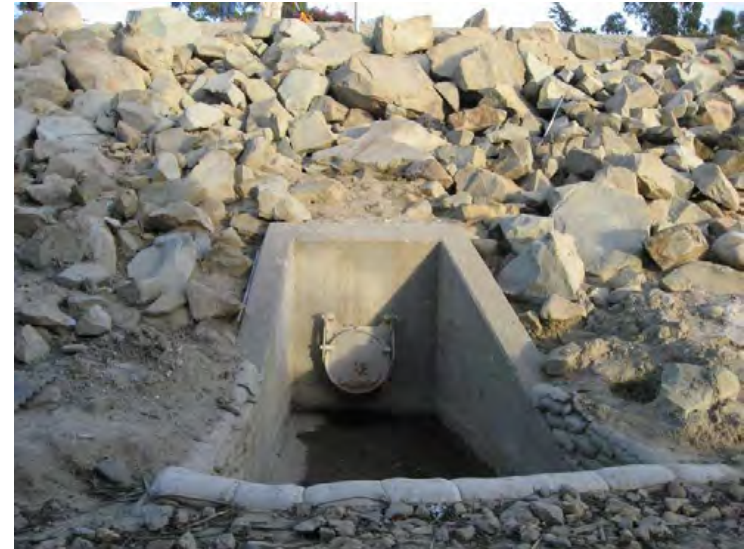
Ventura River Levee, From Ocean to Canada de San Joaquin. (Photo No. P15) - 24" CMP with flap Gate, Peking Drain (riverward side)
