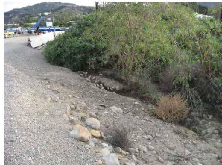
Ventura River Levee, From Ocean to Canada de San Joaquin. (Photo No. M28) – Erosion along levee toe (landward side)
