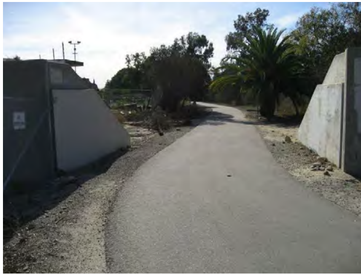
Ventura River Levee, From Ocean to Canada de San Joaquin. (Photo No. P1) - 12 beam stop log system at bicycle path crossing (riverward side)
