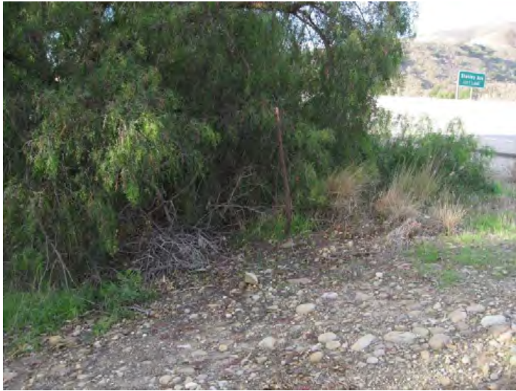
Ventura River Levee, From Ocean to Canada de San Joaquin. (Photo No. M9) - Vegetation within 15' of levee toe, looking d/s (landward side)
