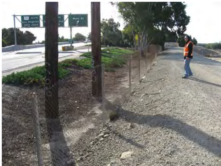
Ventura River Levee, From Ocean to Canada de San Joaquin. (Photo No. M26) – Power poles within 15' of levee toe, looking d/s (landward side)
