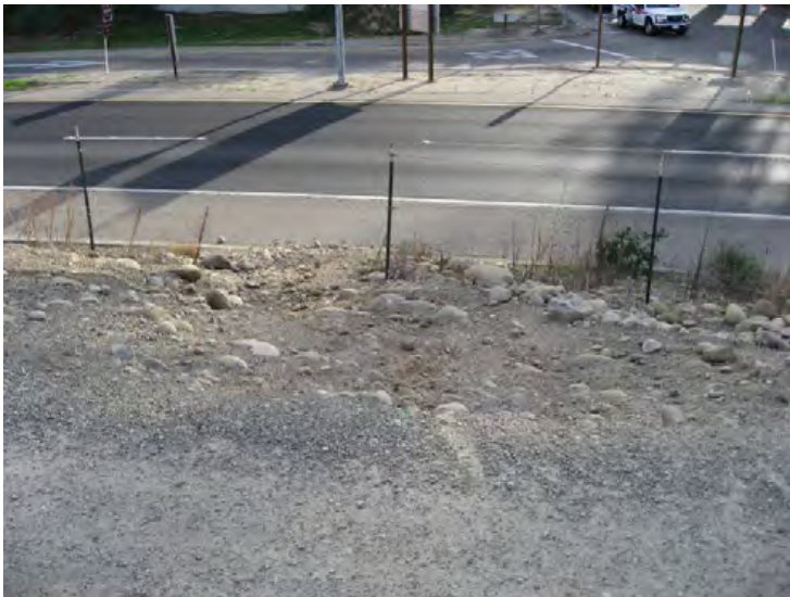
Ventura River Levee, From Ocean to Canada de San Joaquin. (Photo No. M10) - Erosion on levee top and embankment (landward side)
