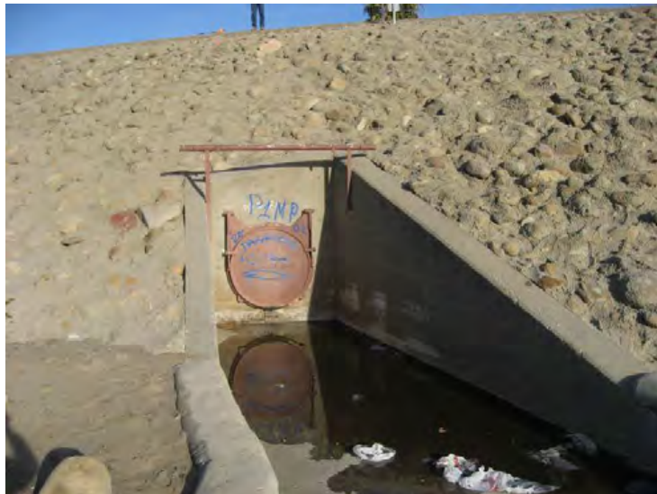
Ventura River Levee, From Ocean to Canada de San Joaquin. (Photo No. P10) - 48" CMP with flap gate, FWY #2 Drain (riverward side)
