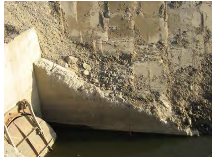
Ventura River Levee, From Ocean to Canada de San Joaquin. (Photo No. M4) - Damaged concrete on headwall with flap gate stuck open (riverward)
