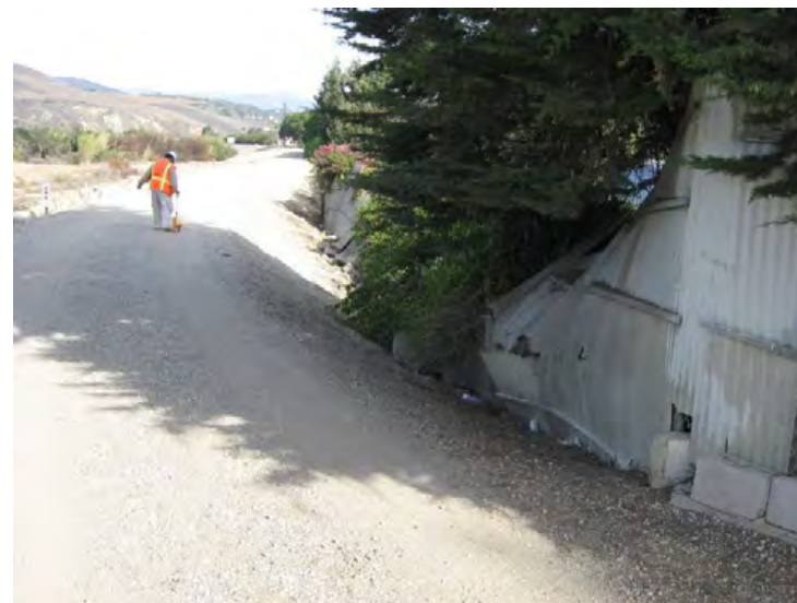
Ventura River Levee, From Ocean to Canada de San Joaquin. (Photo No. M16) - Vegetation within 15' of levee toe, looking u/s (landward side)
