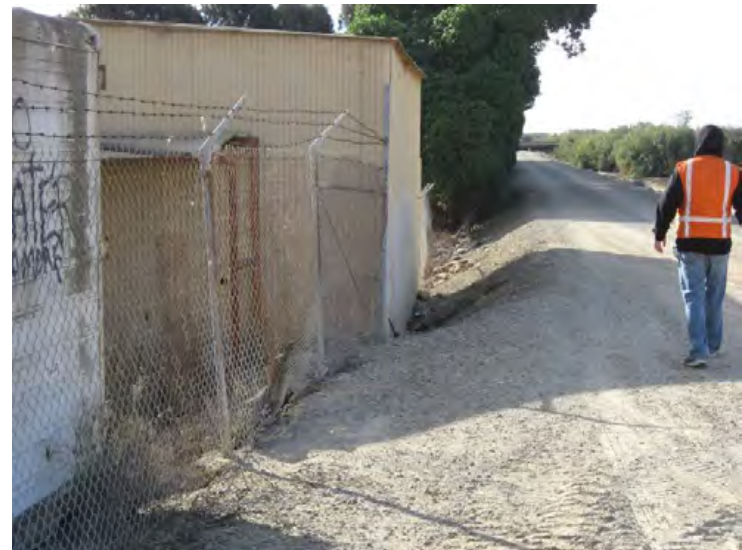
Ventura River Levee, From Ocean to Canada de San Joaquin. (Photo No. M12) - Tin storage shed and miscellaneous debris at levee toe (landward)
