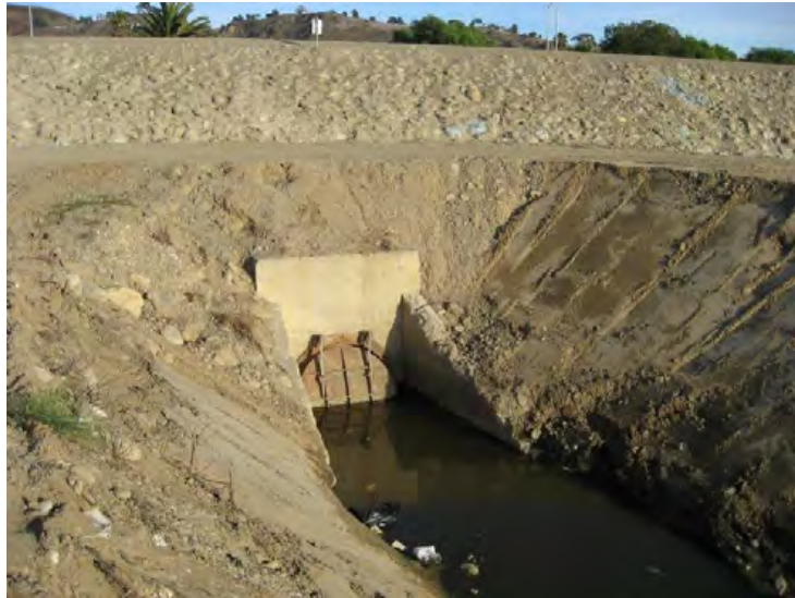
Ventura River Levee, From Ocean to Canada de San Joaquin. (Photo No. P13) - 48" pipe with flap gate, Simpson Drain (riverward side)
