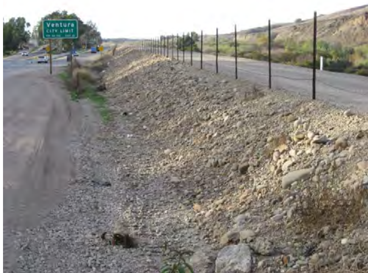
Ventura River Levee, From Ocean to Canada de San Joaquin. (Photo No. F5) – Looking downstream at levee embankment & toe (landward side)
