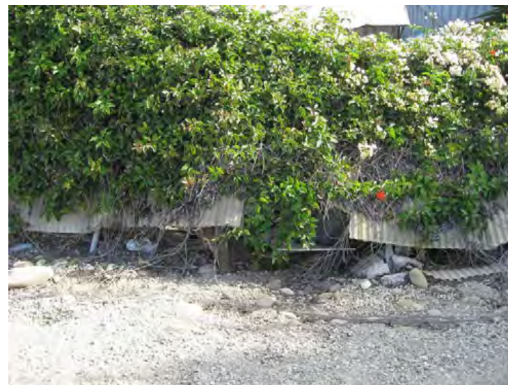
Ventura River Levee, From Ocean to Canada de San Joaquin. (Photo No. M15) - Vegetation within 15' of levee toe (landward side)
