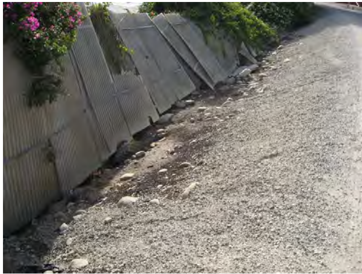
Ventura River Levee, From Ocean to Canada de San Joaquin. (Photo No. M17) – Levee toe has been undercut (landward side)
