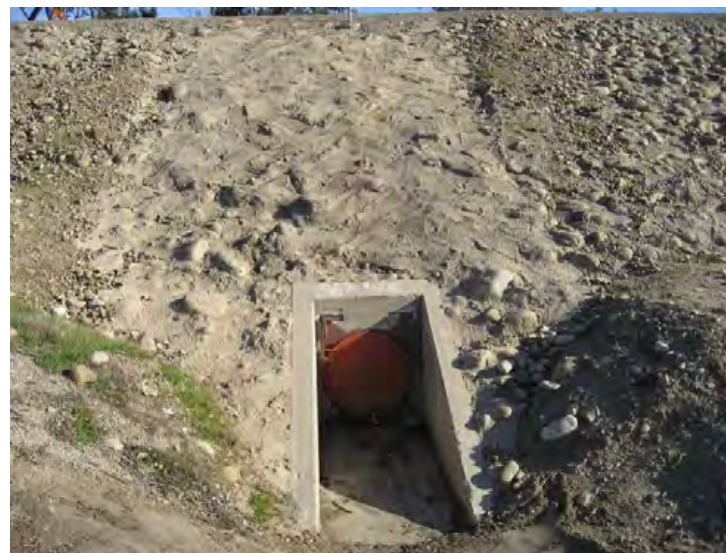
Ventura River Levee, From Ocean to Canada de San Joaquin. (Photo No. P7) - 36" Flap Gate, FWY #4 Drain (riverward side)
