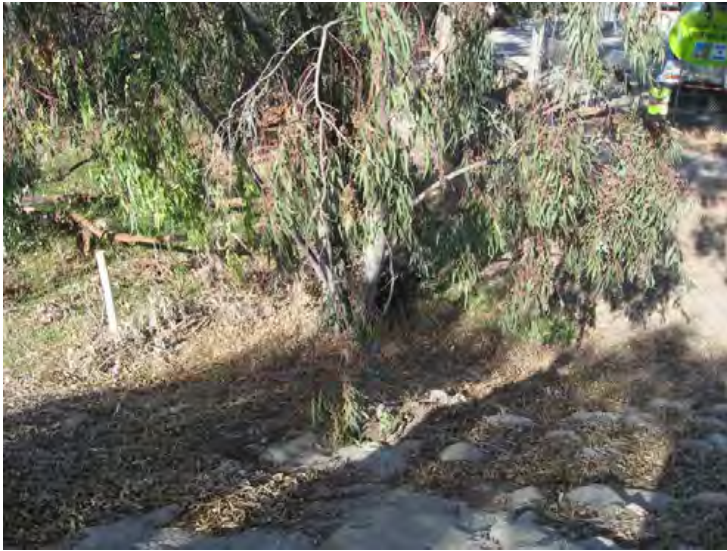
Ventura River Levee, From Ocean to Canada de San Joaquin. (Photo No. M1) - Vegetation within 15' of levee toe (riverward side)
