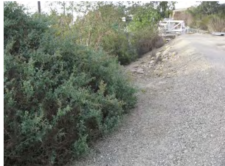
Ventura River Levee, From Ocean to Canada de San Joaquin. (Photo No. M8) - Vegetation within 15' of levee toe, looking d/s (landward side)
