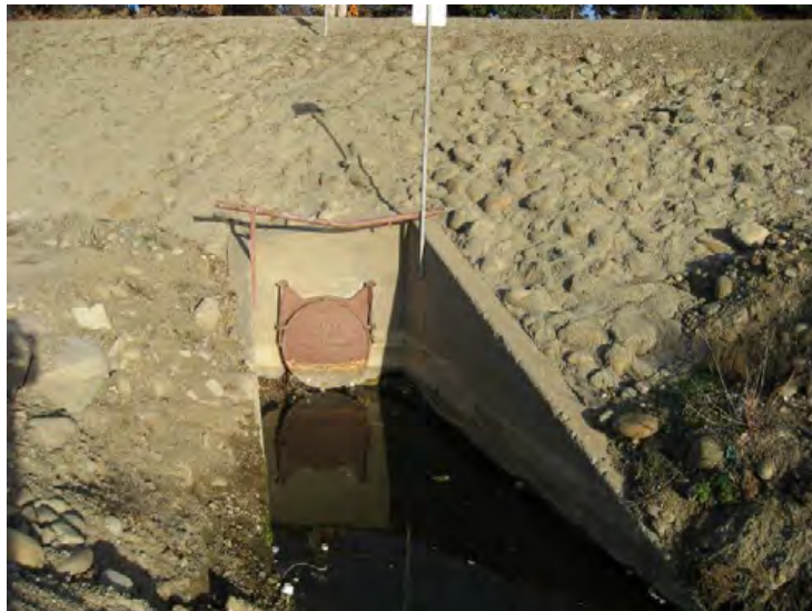
Ventura River Levee, From Ocean to Canada de San Joaquin. (Photo No. P14) - 48" CMP with flap gate, Harrison Drain (riverward side)
