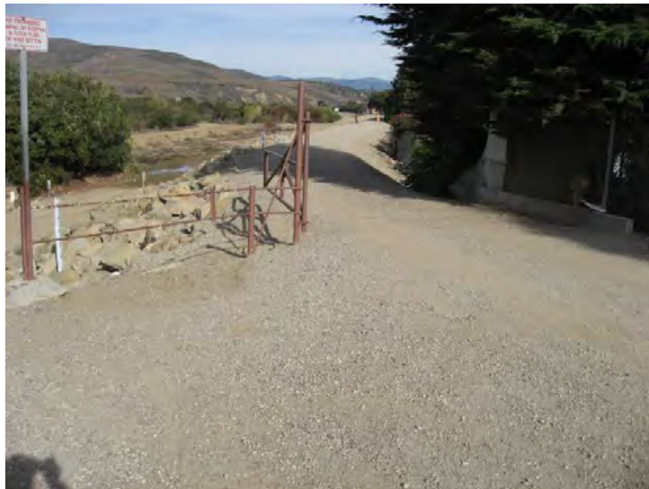
Ventura River Levee, From Ocean to Canada de San Joaquin. (Photo No. M18) - Vegetation within 15' of levee toe, looking d/s (riverward side)
