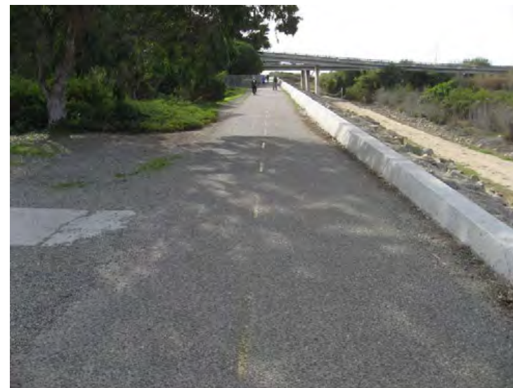
Ventura River Levee, From Ocean to Canada de San Joaquin. (Photo No. F8) – Looking d/s at bike path and flood wall on top of levee
