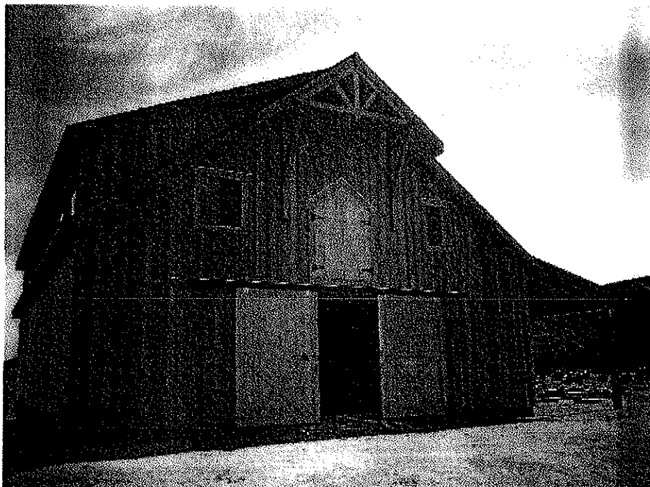
West Side of Barn
