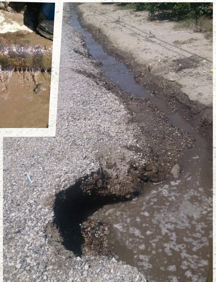
Photos above show a 6” waterline break that occurred in Somis (WWD19).
